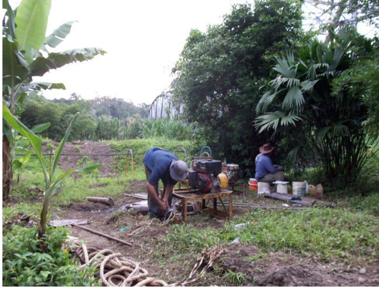
Photo 7: View of the site of Río Estrella Bridge where the borehole was executed. The borehole is on the right margin of the river. Notice the bridge to the right.
