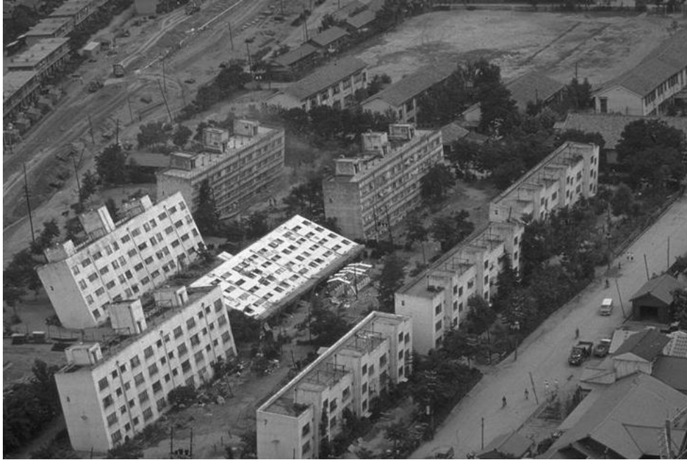
Figure 2-14: Bearing Capacity Failures Following 1964 Niigata, Japan Earthquake (Courtesy of EERC, Univ. of Calif.)
