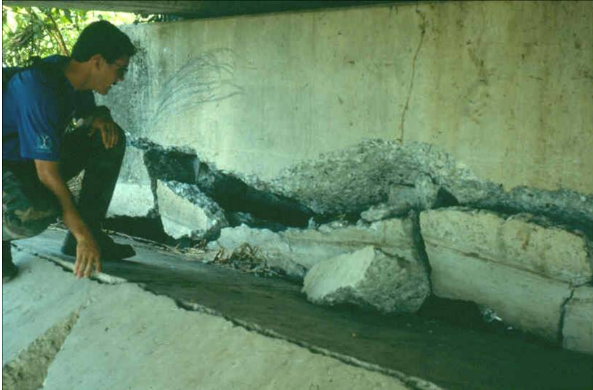
Figure 10-2: Rotated Pile Cap at the South Abutment of the Rio Bananito Highway Bridge
