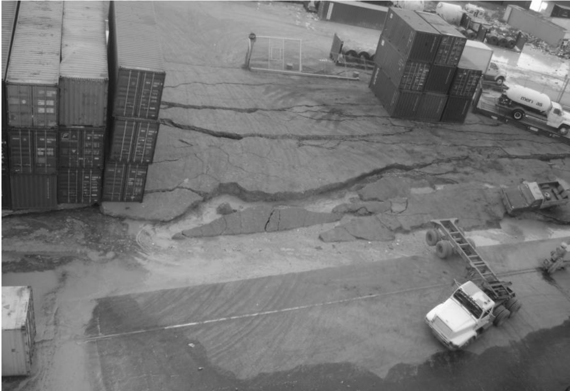
Figure 2-17: Lateral Spread at the Port in Port-au-Prince, Haiti Following the 2010 Earthquake (Courtesy of EERI)
