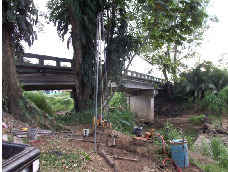
Photo 2: View of the site of Río Blanco Bridge where the borehole was executed. The borehole is on the right margin of the river.
