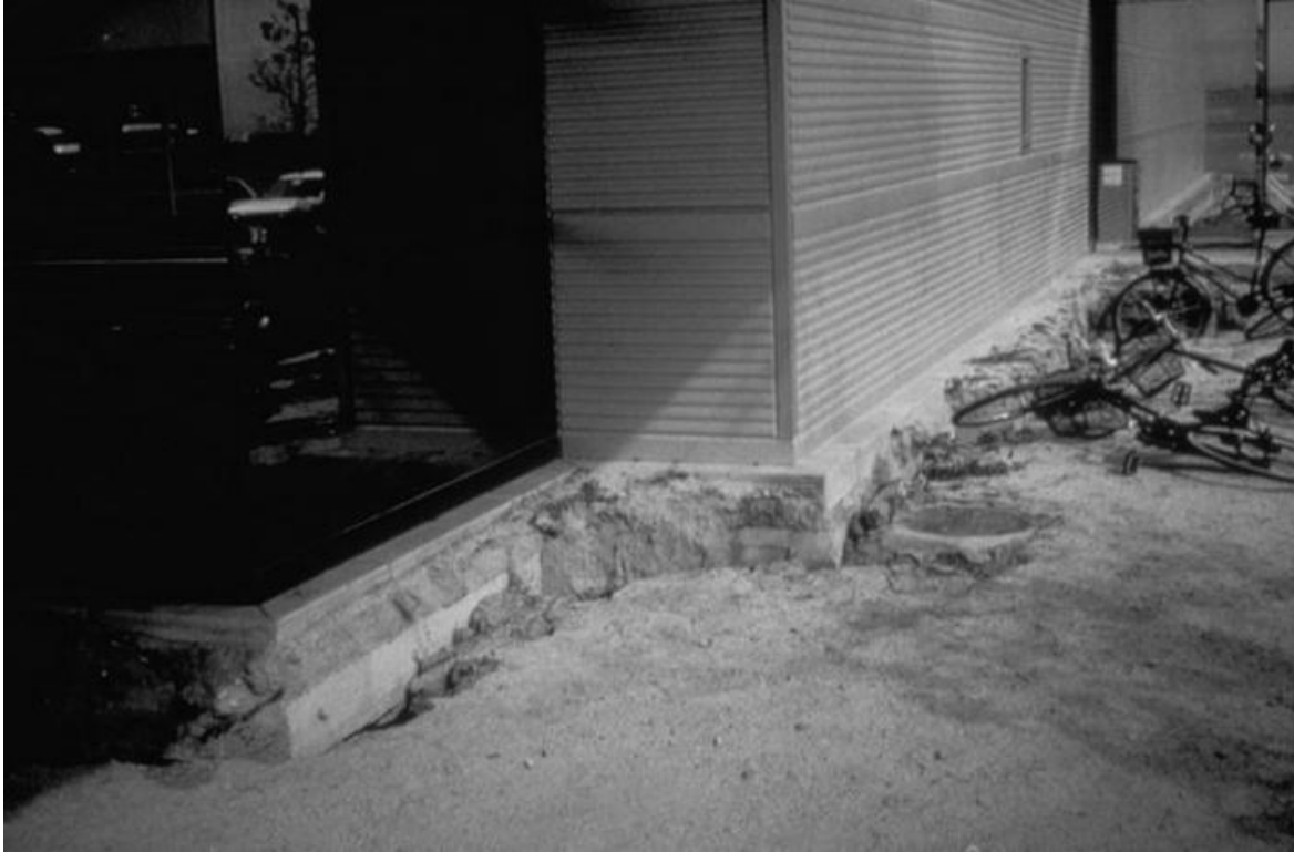
Figure 2-13: Settlement Around a Structure in Kobe, Japan Following 1995 Hyogoken-Nanbu Earthquake (Courtesy of EERC, Univ. of Calif.)
