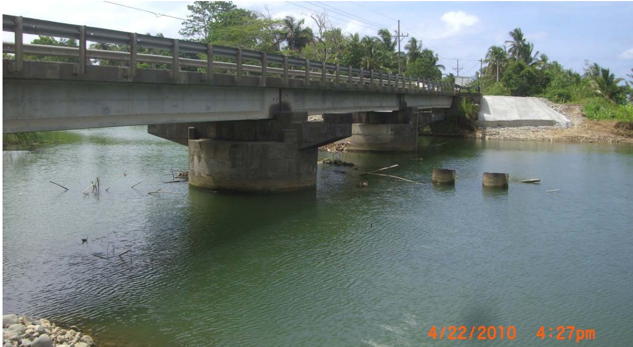
Figure 10-1: The Current Rio Bananito Highway Bridge
